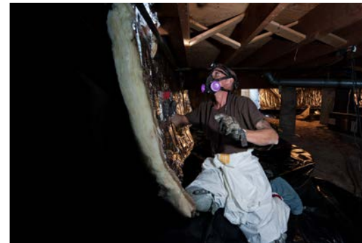
Installing crawlspace insulation.
