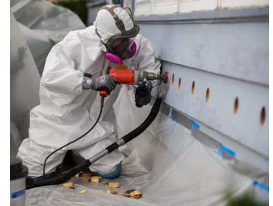
Installing exterior insulation.
