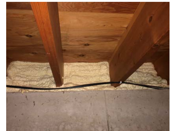
Rim joist installation.
