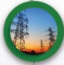
Transmission and Distribution Infrastructure
