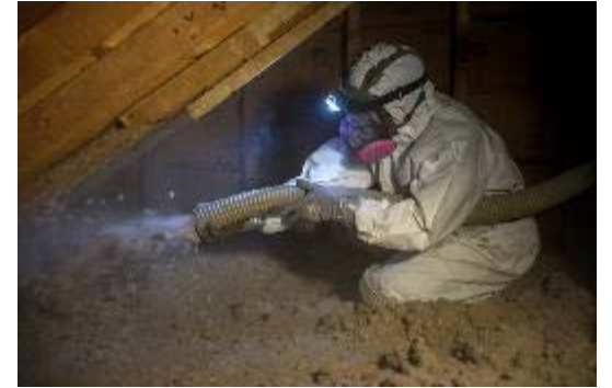
Installing attic insulation. Image by Dennis Schroeder, NREL 28694
