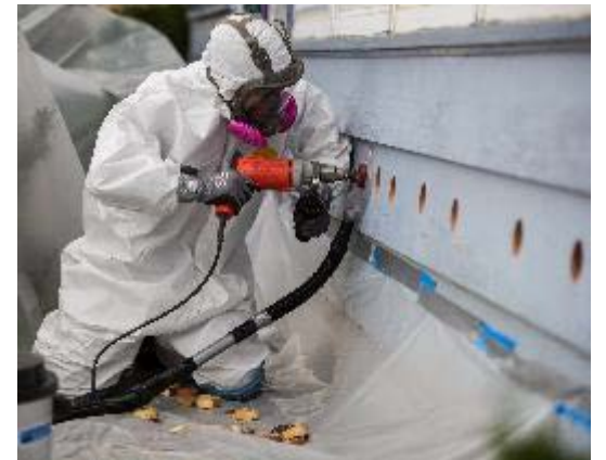
Installing exterior insulation. Image by Dennis Schroeder, NREL 28725
