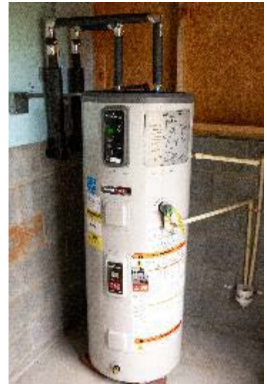
Heat Pump Water Heater. Image from Habitat for Humanity of Catawba Valley, via Building America Solution Center
