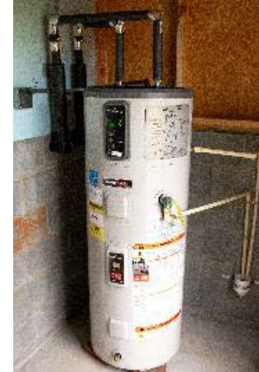
Heat pump water heater. Image from Building America Solution Center
