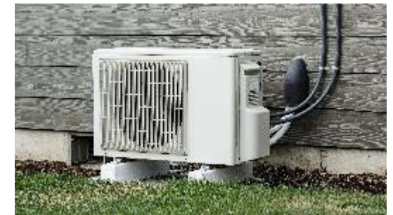
Heat pump outside compressor. Image from Building America Solution Center
