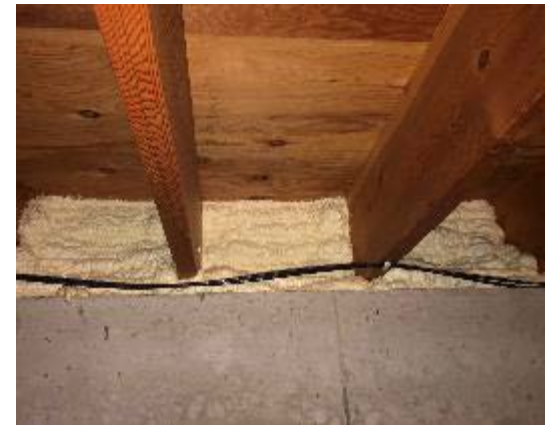
Rim joist installation. Image by Corry Chovanec, NREL
