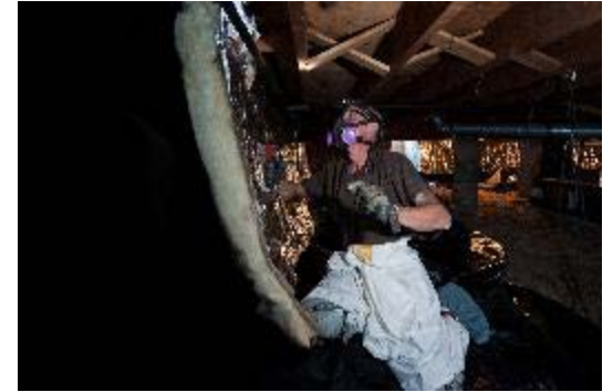
Installing crawlspace insulation. Image by Dennis Schroeder, NREL 17972.
