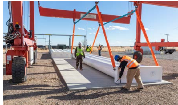
Installing hydrogen storage at ARIES. Photo by Werner Slocum, NREL
