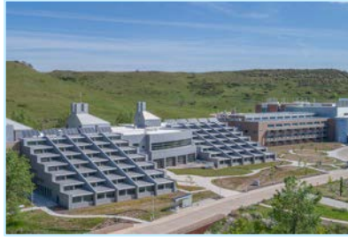
Solar Energy Research Facility Science and Technology Facility Field Test Laboratory Building
