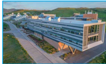
Energy Systems Integration Facility
