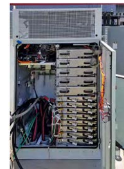
Vendor 3: 125 kW building block w/ HF isolation – only up to 500 V
