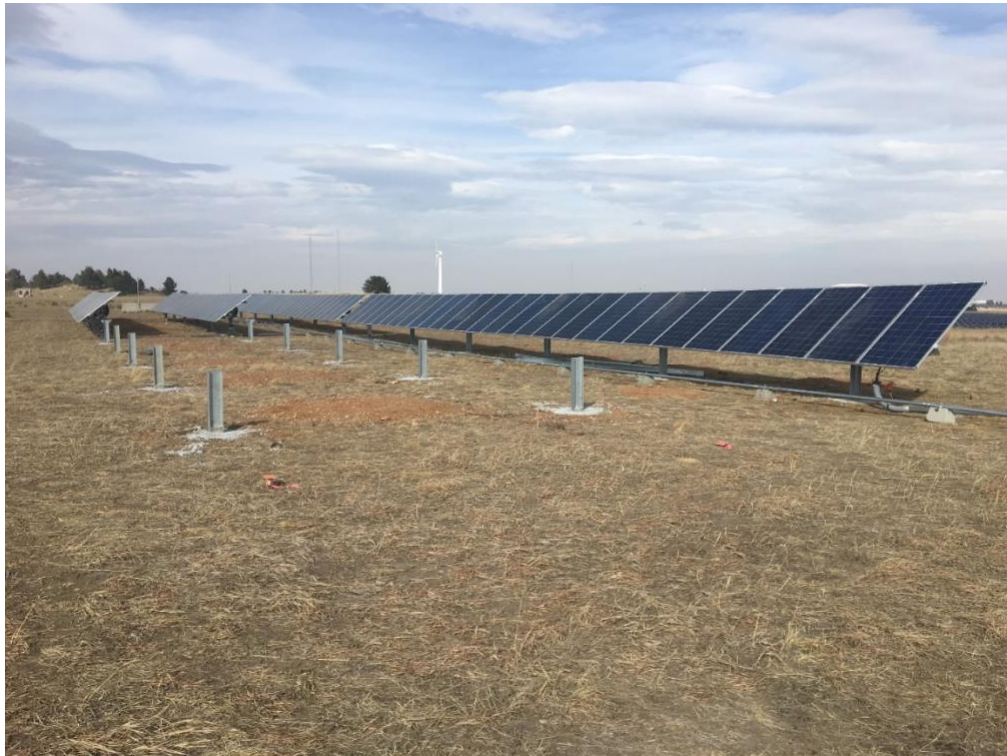
Figure 2. Initial array installation
