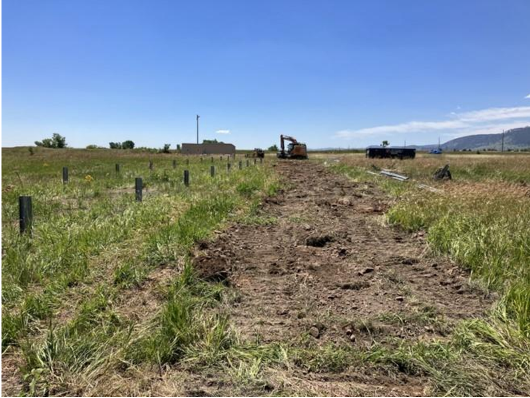
Figure 15. Excavator working on pier removal
