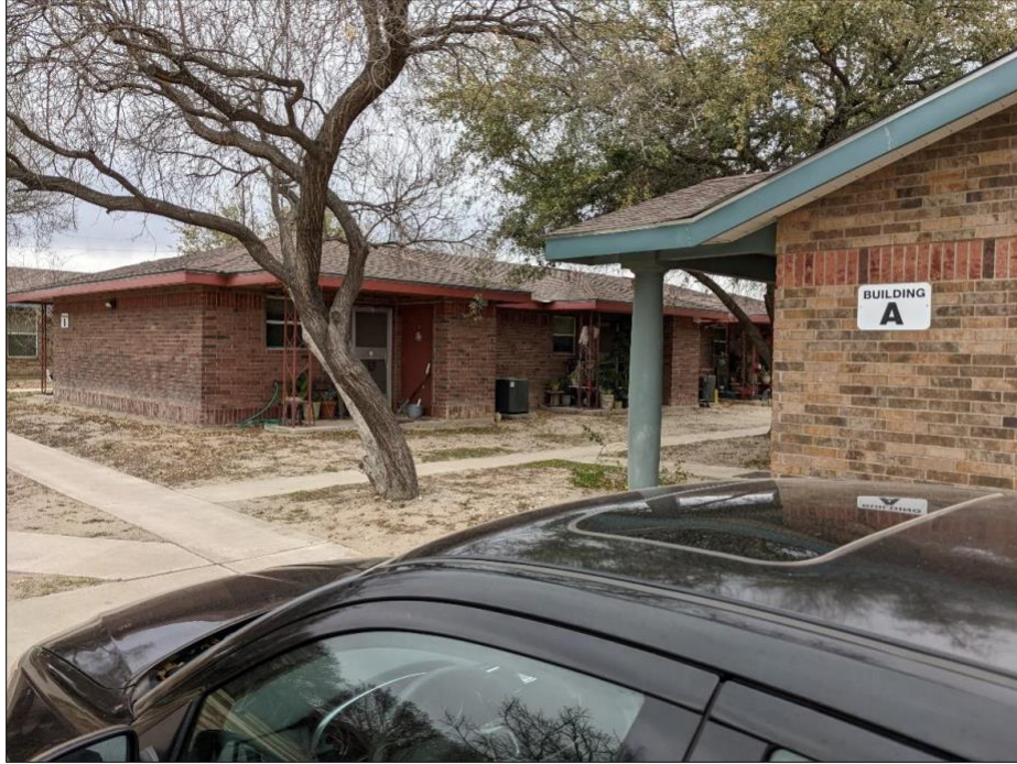
Figure 3. Buildings A and B from the parking lot.
