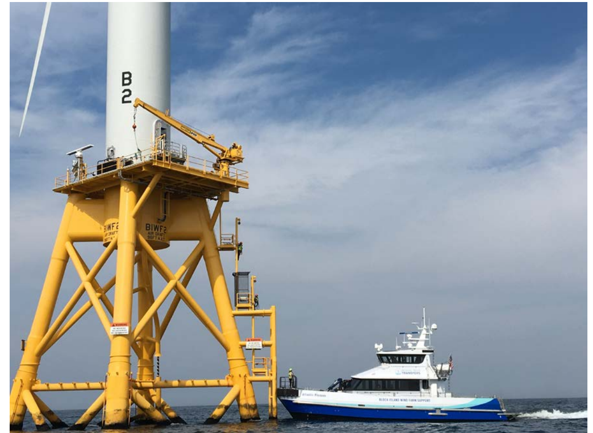
Figure. Offshore wind turbine service vessel
