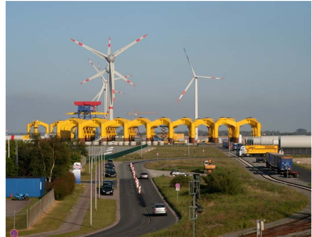
Figure. Foundations at an offshore wind marshalling port
