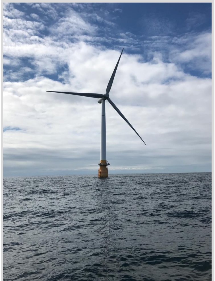
Using FAST.Farm software, NREL researchers studied wake dynamics on floating offshore wind turbines, like the one shown here. The results will have growing importance as floating offshore wind energy advances. Photo by Brent Rice, NREL 52798
