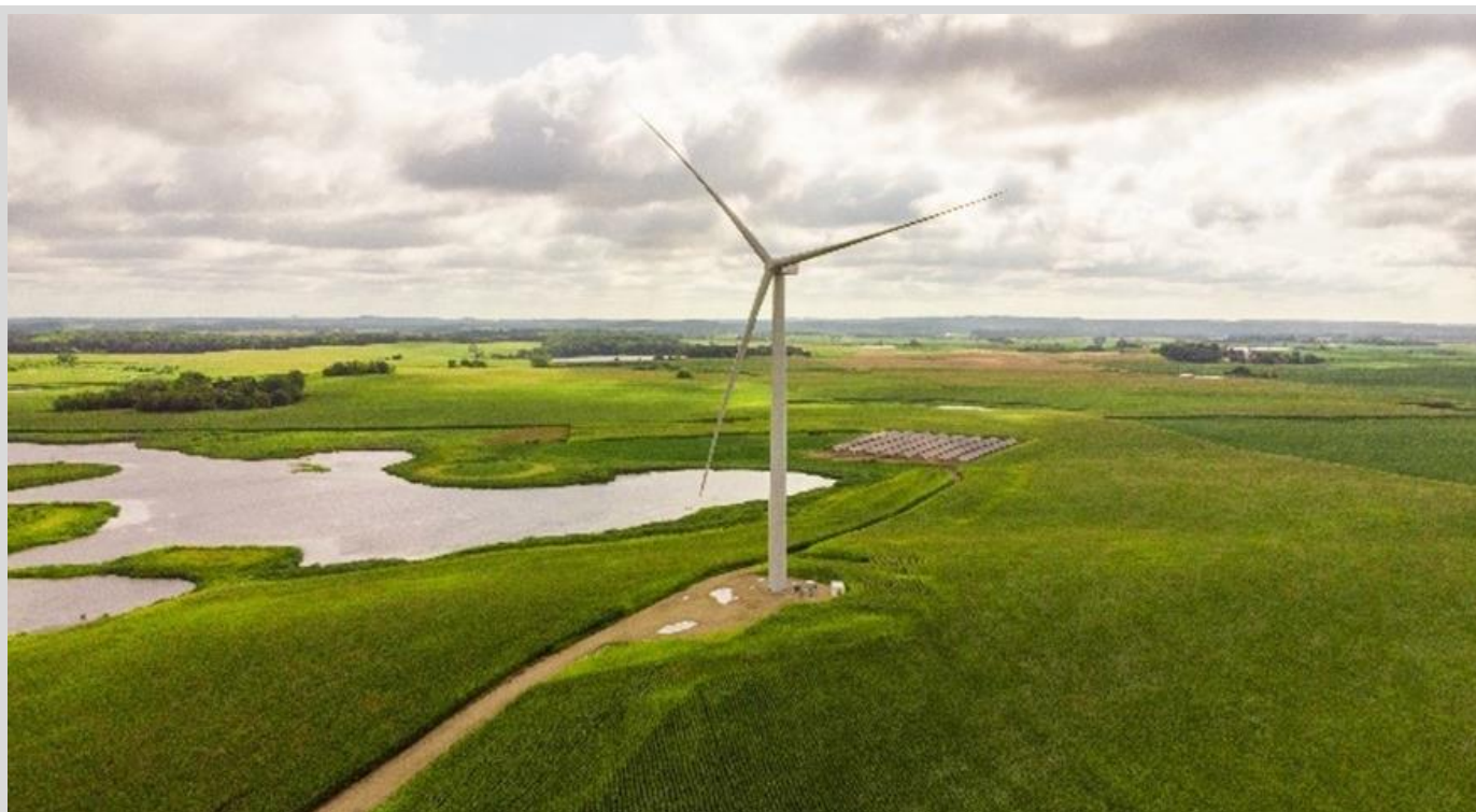
Two new resources—a national network and resource hub—are designed to provide comprehensive information, tools, and support to anyone interested in deploying distributed wind turbines, like this 2.3-MW turbine that, along with a nearby 500-kilowatt solar photovoltaic array, provides power to a Minnesota electric cooperative. Photo from Lake Region Electric Cooperative
