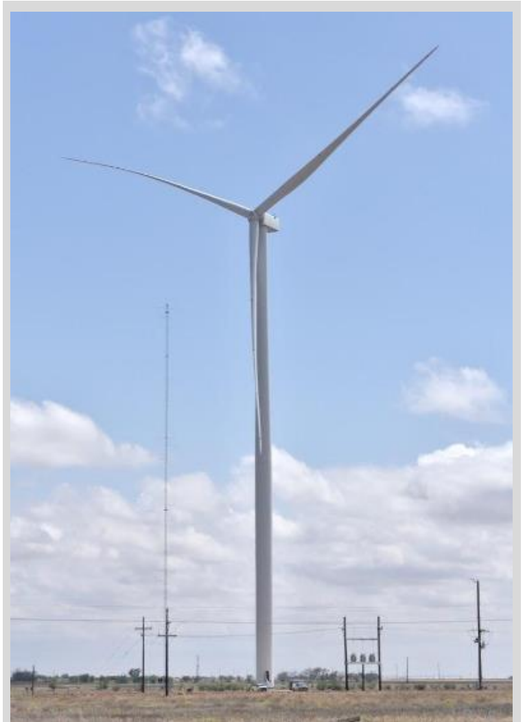
NREL researchers used the now-decommissioned GE 2.8-MW wind turbine to characterize structural damping of modern wind turbine blades. Photo from GE Vernova
