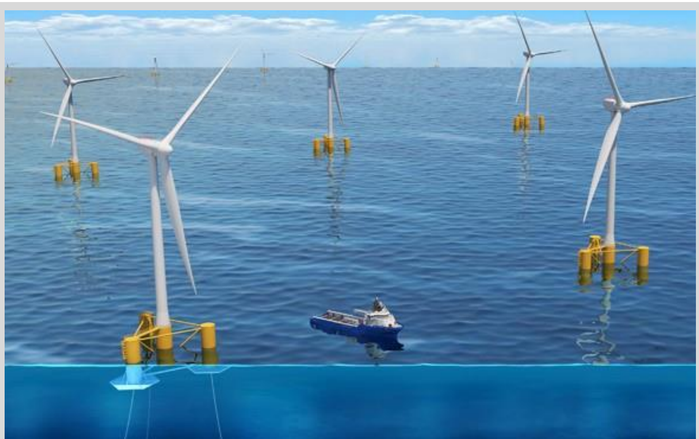
IEA Wind’s Offshore Code Comparison Collaboration 7 project brings together over 100 industry leaders to refine offshore wind energy design modeling tools, with a focus on advancing floating offshore wind structures, like the ones shown here. Image by Besiki Kazaishvili, NREL
