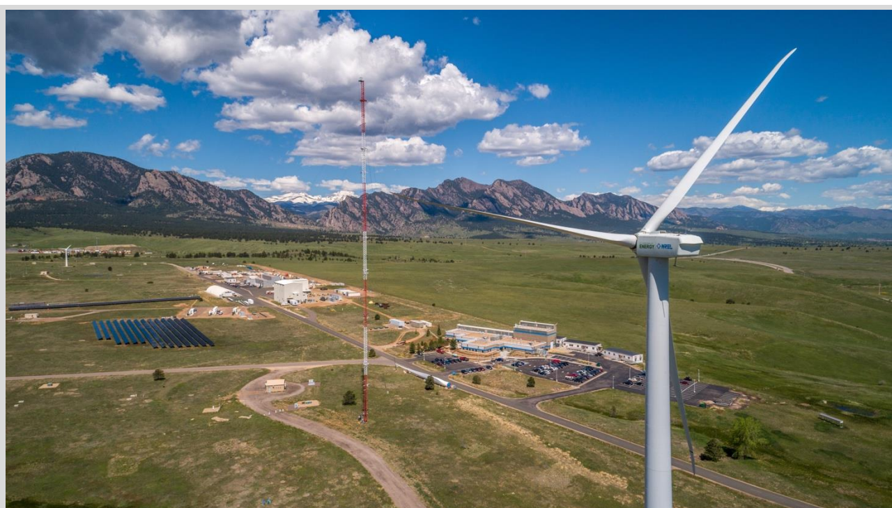
NREL's new wind turbine, capable of generating 3 MW and more, will provide a more current wind energy research platform than the General Electric 1.5-MW turbine, shown here, whose design is more than 20 years old. Photo by Josh Bauer, NREL 61829
