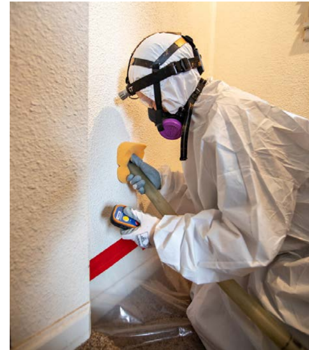
Photo by Werner Slocum, NREL 72235
