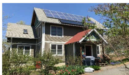
Residential rooftop solar (about 10 kW on one roof, enough to power 1 home)
