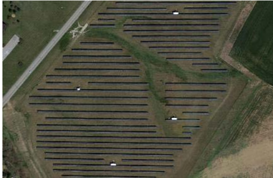
Inverters are exposed & easily visible
