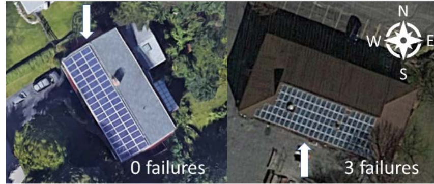
Arrow points out inverter location
