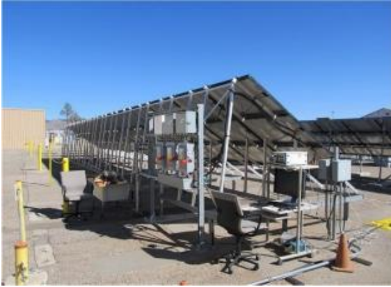
Test set-up used at DETL of SNL
