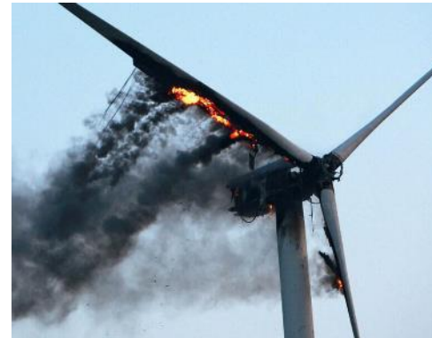
Wind turbine at fire due to failed IGBT module 1
