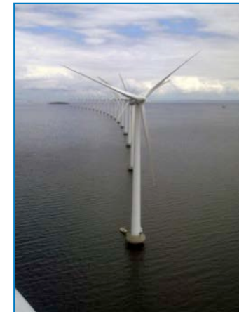
Photo from HC Sorensen, NREL 17855
