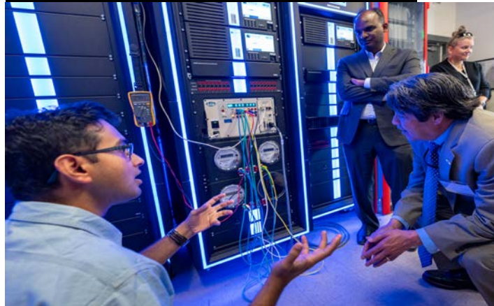
Photo by Werner Slocum | NREL 78586
