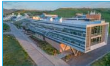
Energy Systems Integration Facility
