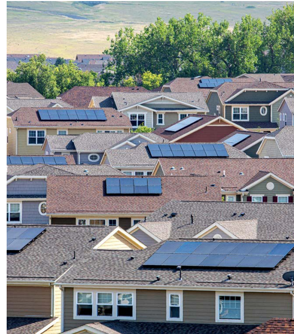
Photo by Werner Slocum, NREL 66338
