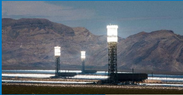
Ivanpah CSP Plant in California NREL image 46269 Direct steam power tower → no storage!
