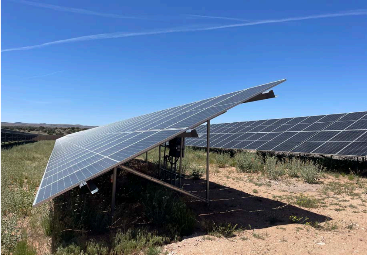
Example of a south facing fixed-tilt solar array (Photo credit: Laura Beshilas, NREL)
