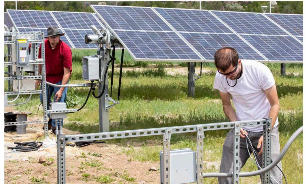
Ongoing maintenance at an agrivoltaics array (Photo credit: Werner Slocum, NREL)
