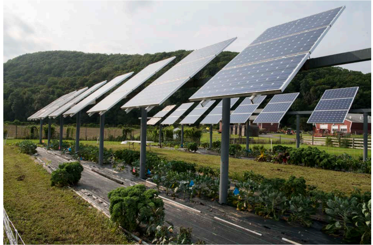
Vegetables grow under solar panels at a test plot at the UMass Crop Animal Research and Education Center in South Deerfield, MA. (Photo credit: Dennis Schroeder, NREL)
