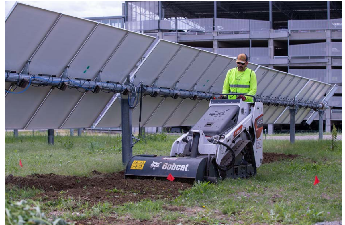
Tilling of the soil at a monofacial agrivoltaic array (Photo credit: Joe DeINero, NREL)
