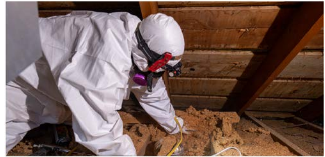
Air Sealing an Insulation-Contact Rated Fixture (2)
