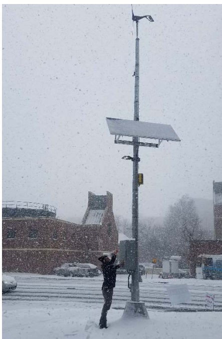
Figure 2. Micro wind turbine from Primus Windpower (now Ryse Energy) providing data for educational purposes at Appalachian State University. Photo by Brent Summerville, National Renewable Energy Laboratory (NREL)
