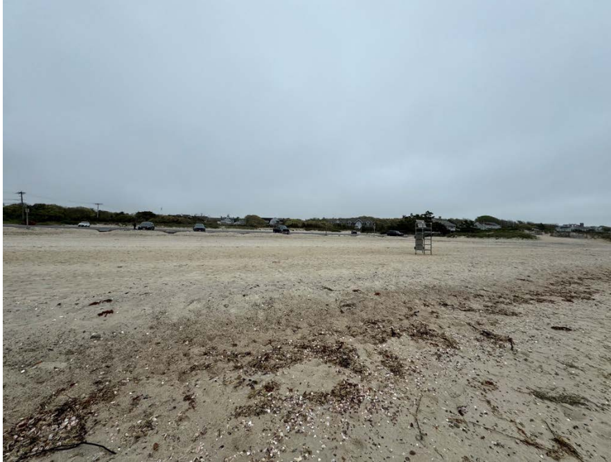
Figure 30. Covell's Beach in Barnstable, Massachusetts, is the location of the cable landing site for the Vineyard Wind 1 project. This photo was taken in May 2024, following completion of the cable installation and restoration of the beach and parking lot. Photo from Mary Ann Labue
