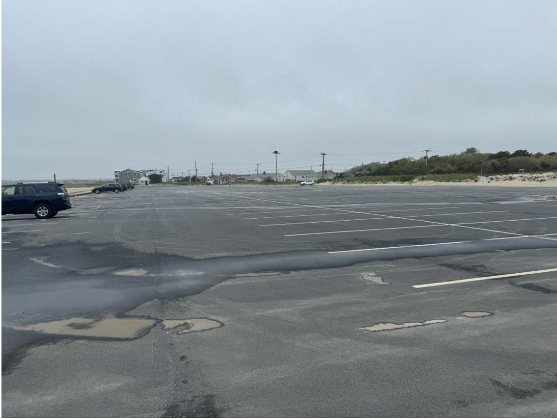
Figure 26. The parking lot at Covell's Beach in Barnstable, Massachusetts, in May 2024, after construction of the underground cable for the Vineyard Wind 1 project was completed and the area was restored to previous conditions. Photo from Mary Ann Labue
