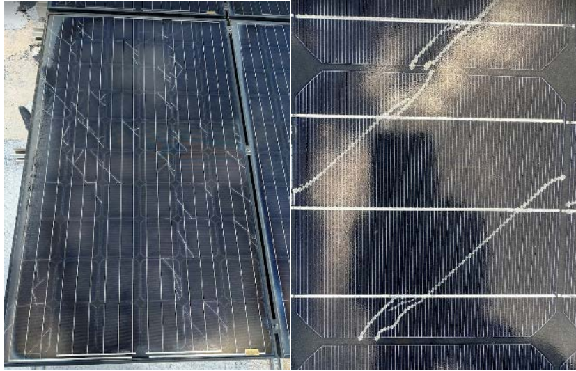
Figure 59. Snail trails most likely predated the storm, though they can be caused by water ingress. These will lead to loss of production over time and may be grounds for a warranty claim.
