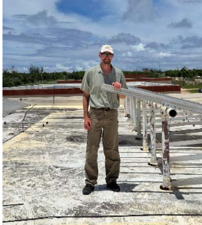
Figure 41. PV racking with high tilt angles allows more wind uplift forces on the undersides of the modules
