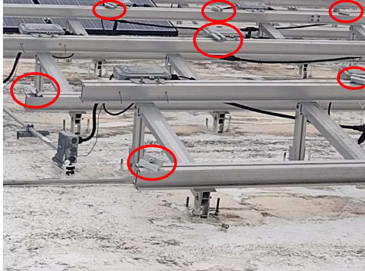
Figure A-7. Clamps largely still present in racking even after modules dislodged
