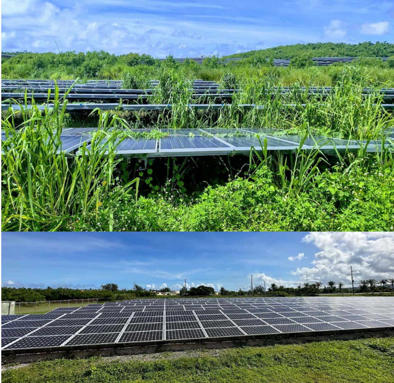
Figure 61. Vegetation management is a big concern on Guam. Top: An overgrown section of a utility-scale PV array. Bottom: An excellently maintained PV array at Naval Base Guam. There is a third-party service contract for this array, and it is in excellent condition, even 15 years after installation.
