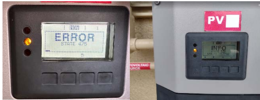
Figure 57. Inverter error codes. Many inverters displayed error codes and were not providing power, even before the storm.
