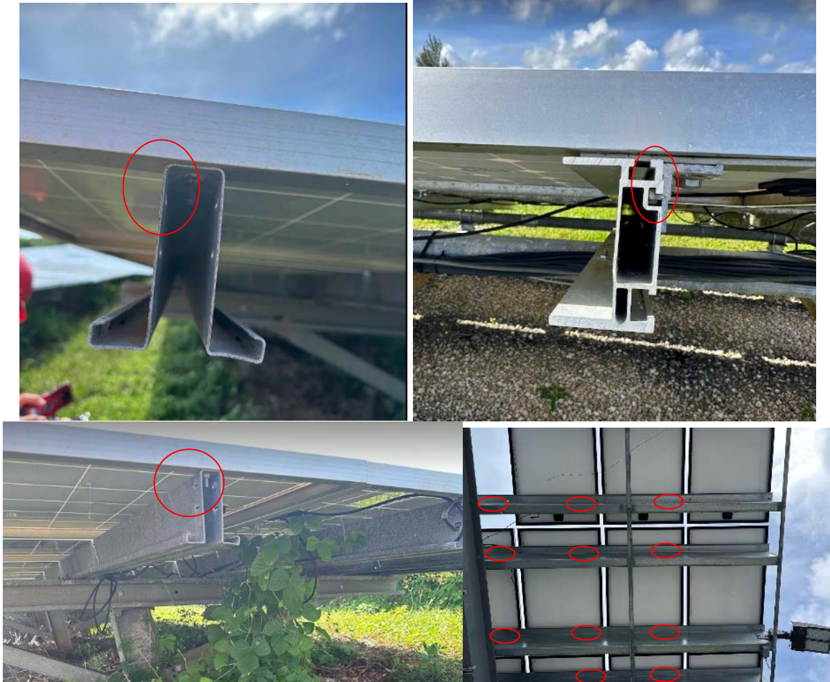
Figure 31. Various through-bolting approaches in which the bottom flange of the module's metal frame is bolted directly to the racking system underneath
