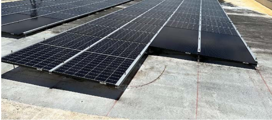
Figure 22. One local racking system utilizes a continuous clamping approach down the entire length of the modules
