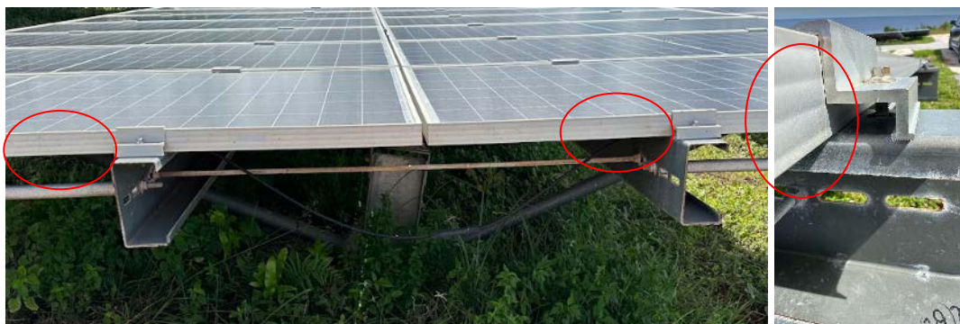
Figure 26. Top clamps through-bolted directly to racking rails are more secure because they cannot rotate out of rail slots
