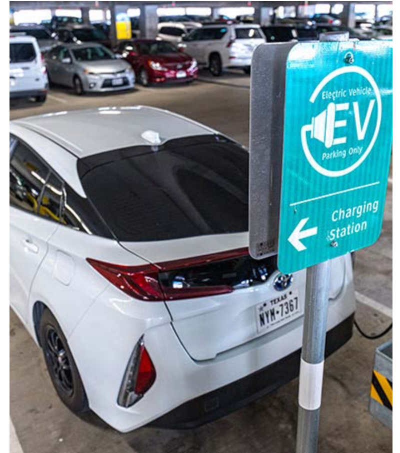
An electric rental car charges at a DFW charging station. Photo by Werner Slocum, NREL
