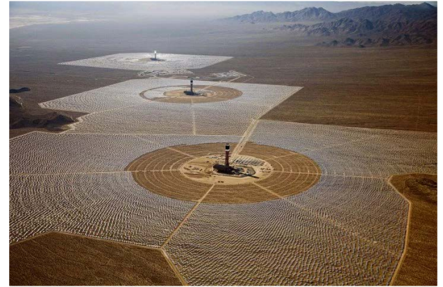
390-MWe Ivanpah Solar Electric Generating Plants
