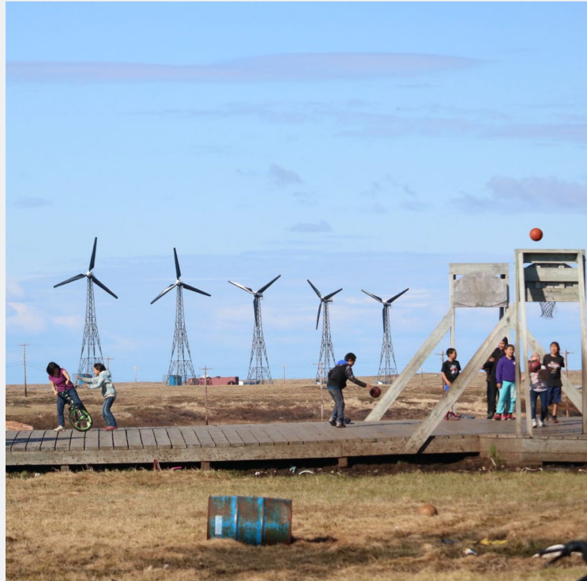
Figure 6. Kongiganak's community wind project. Photo from Amanda Byrd, Alaska Center for Energy and Power
