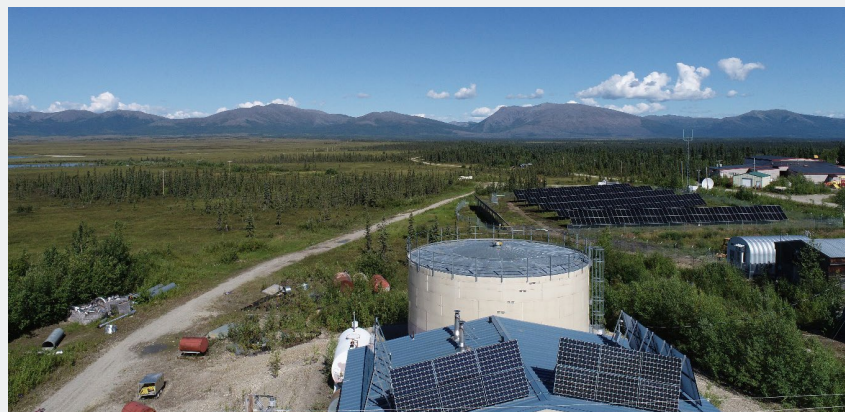
Figure 12. Shungnak's solar PV project, water treatment plant, and water tank. Photo from Alaska Native Tribal Health Consortium
