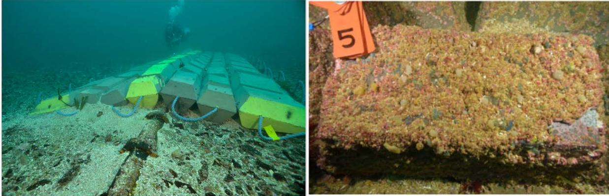
**Figure 11. (left) Newly installed concrete mattress over partially exposed subsea cable. (right) Close-up image of a concrete mattress that has been colonized by organisms after installation.**
