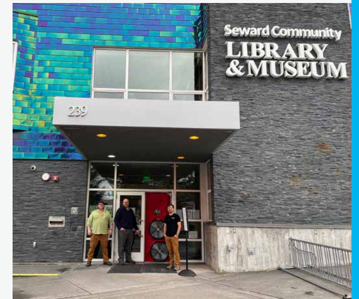
The city of Seward, Alaska, is the location of a new district heat loop project that will provide over 90% of heating and cooling needs for select district buildings by utilizing heat pumps in the basement of the Seward Community Library and Museum. Photo by Matt Mitchell, NREL
