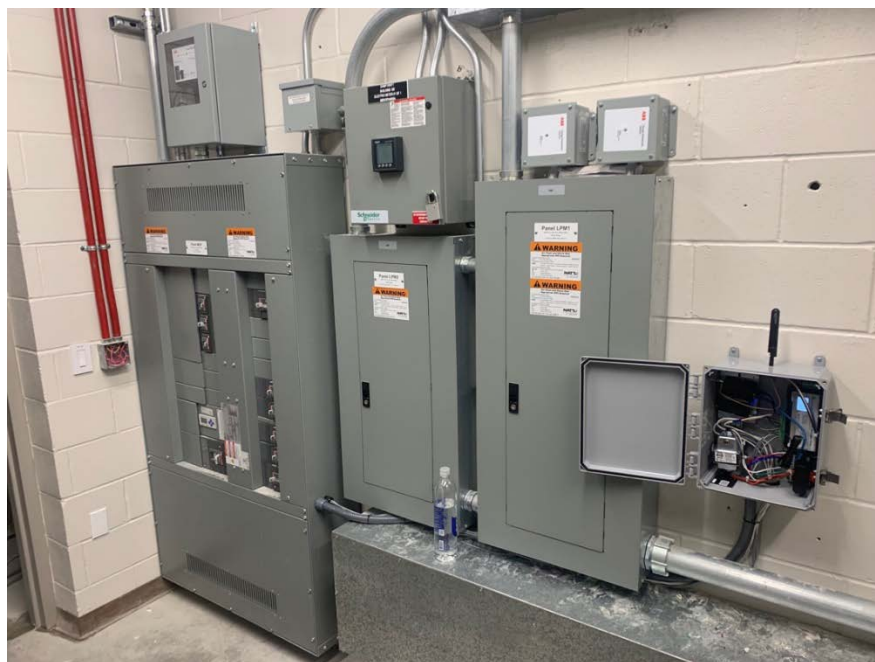
Figure 7. Camp Swift RC with metering installed
