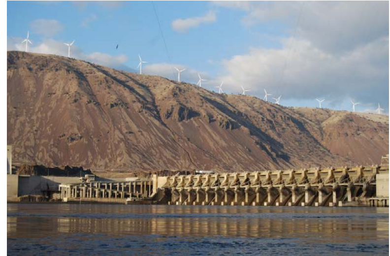
Fig. The ideal clean energy marriage of hydropower and wind power in the Pacific Northwest.
