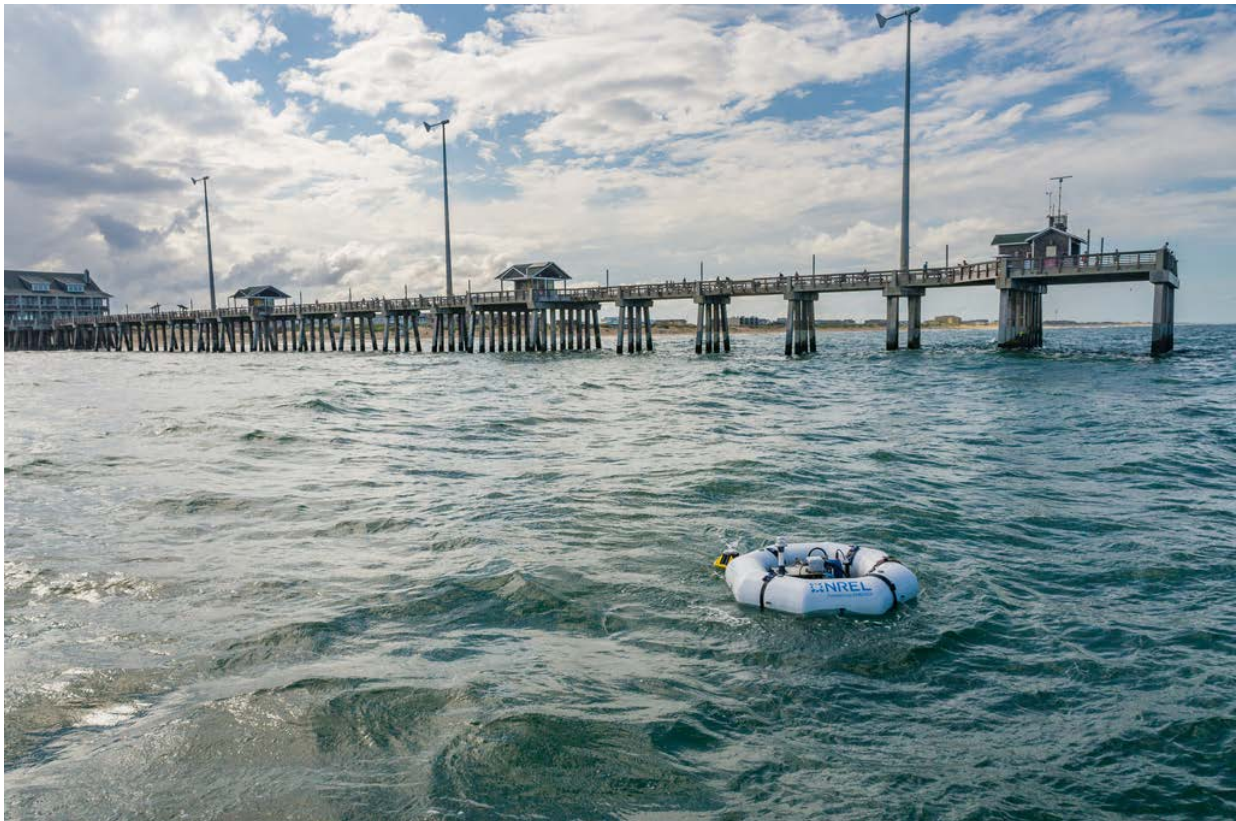
Figure 2. The HERO WEC installed in the ocean, with Jennette's Pier in the background
