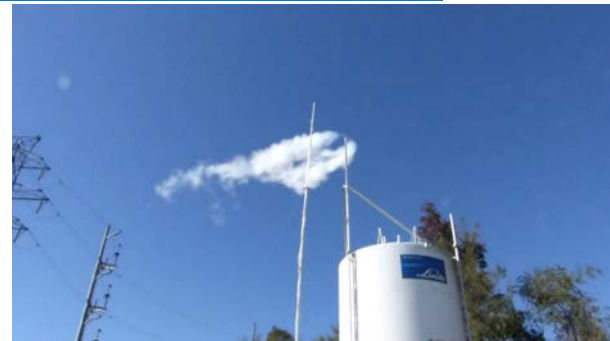
LH2 Venting following delivery
