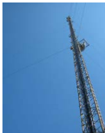
Regional-level tall tower N 2 O
