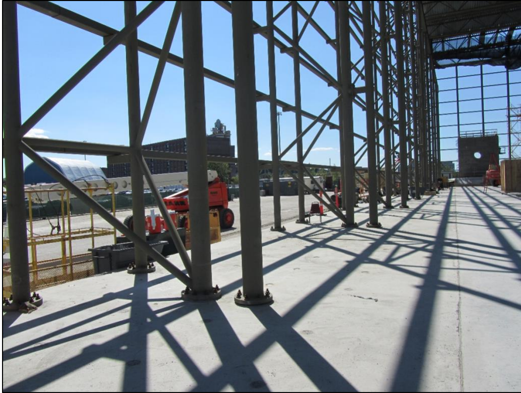
Figure 3 - WTTC wall trusses and test stand (20 August 2010)
