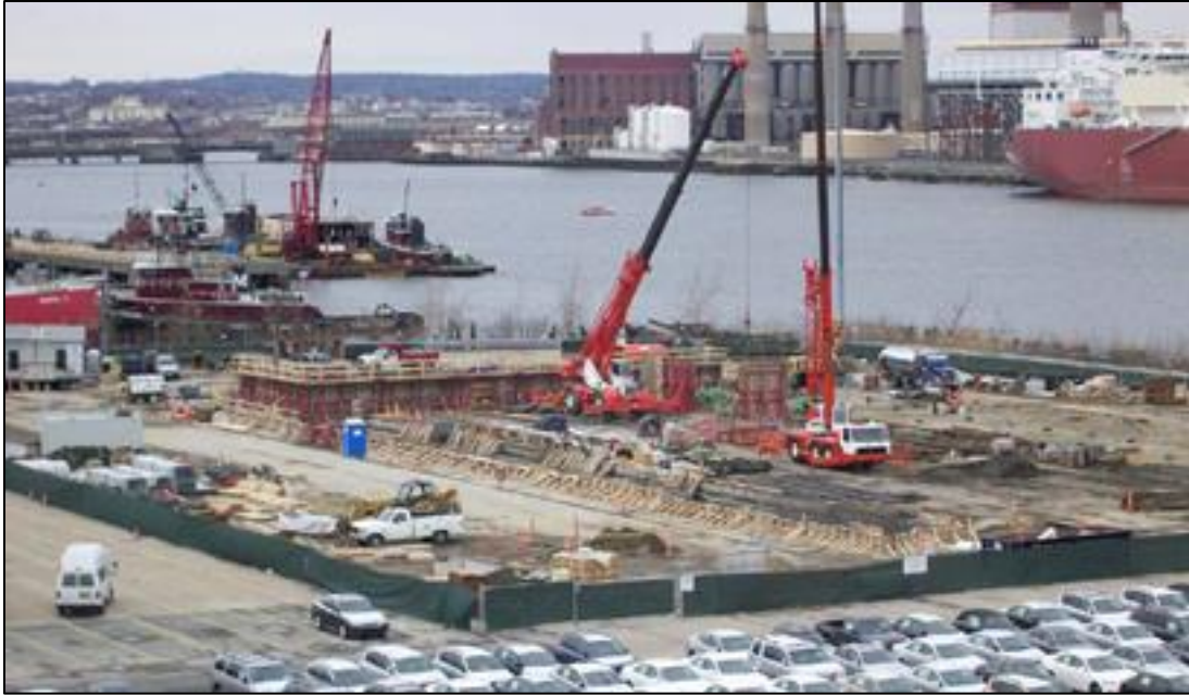
Figure 1 - Pile driving at construction site for the MassCEC WTTC (25 March 2010)
