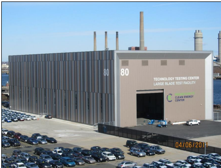
Figure 6 – WTTC Completed Exterior (06 April 2011)
