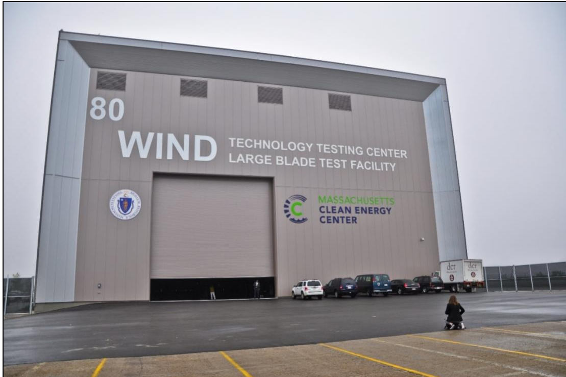
Figure 14 - WTTC Commissioning (18 May 2011)
