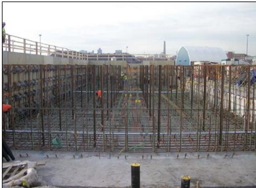
Figure 2 - Rebar placement for the test stand support structure (13 April 2010)
