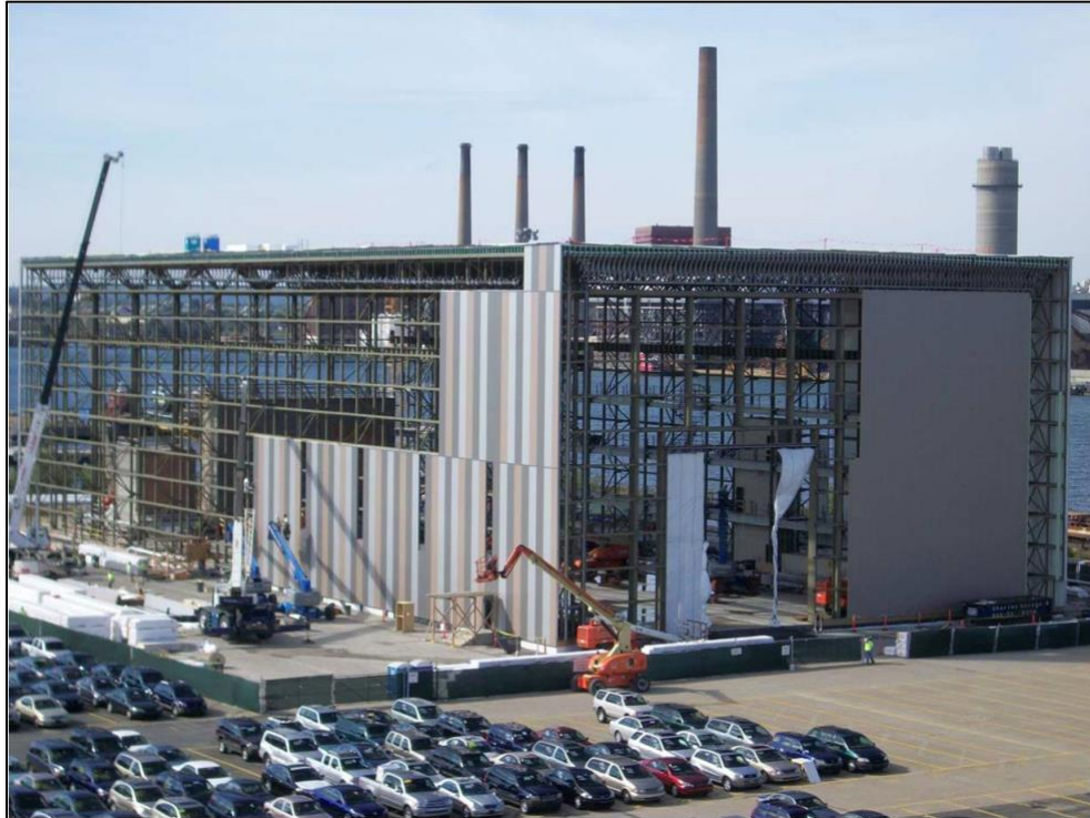
Figure 4 – Application of siding to WTTC (22 February 2011)
