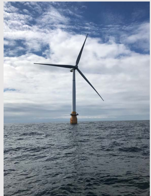
Using FAST.Farm software, NREL researchers studied wake dynamics on floating offshore wind turbines like the one shown here. The results will have growing importance as floating offshore wind energy advances. Photo by Brent Rice, NREL
