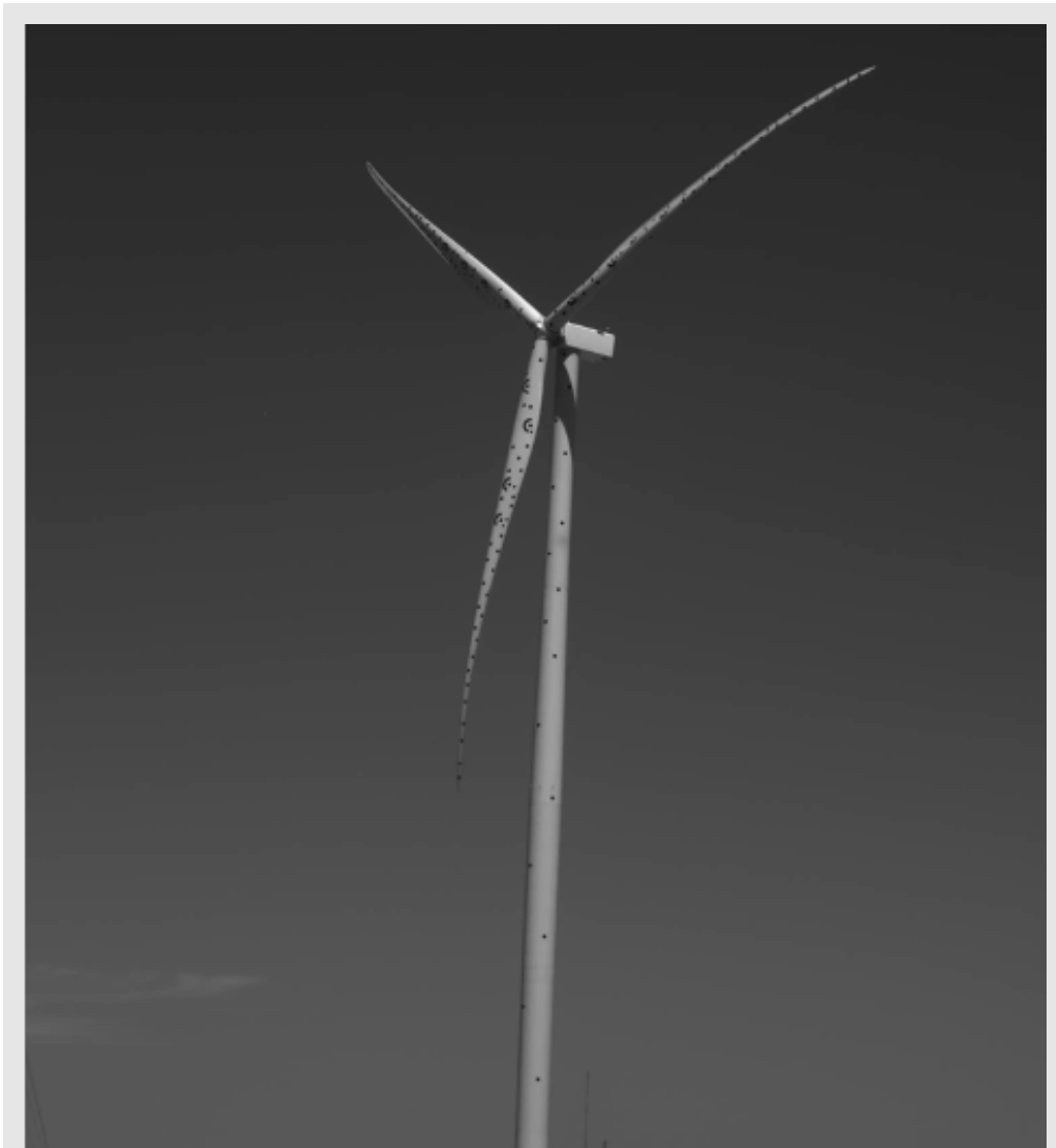
NREL researchers triggered faults on this wind turbine to cause structural loads, resulting in the tower deflection shown here. The markers on the tower and blades were used to measure these motions. Photo by Nicholas Hamilton, NREL
