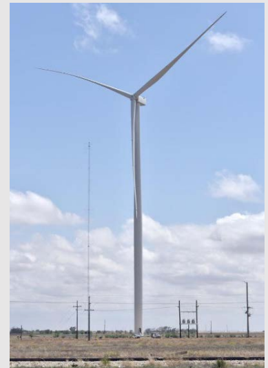
NREL researchers used the now-decommissioned GE 2.8-MW wind turbine to characterize structural dampening of modern wind turbine blades. Photo from GE Vernova
