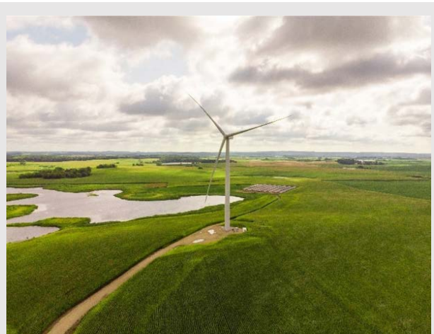
Two new resources—a national network and resource hub—are designed to provide comprehensive information, tools, and support to anyone interested in deploying distributed wind turbines like this 2.3-MW turbine that, along with a nearby 500-kilowatt solar photovoltaic array, provides power to a Minnesota electric cooperative. Photo from Lake Region Electric Cooperative.
