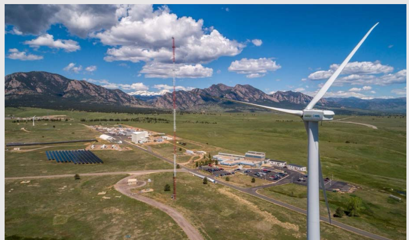
NREL's new wind turbine, capable of generating 3 MW or more, will provide a more current wind energy research platform than the General Electric 1.5-MW turbine, shown here, whose design is more than 20 years old. Photo by Josh Bauer, NREL
