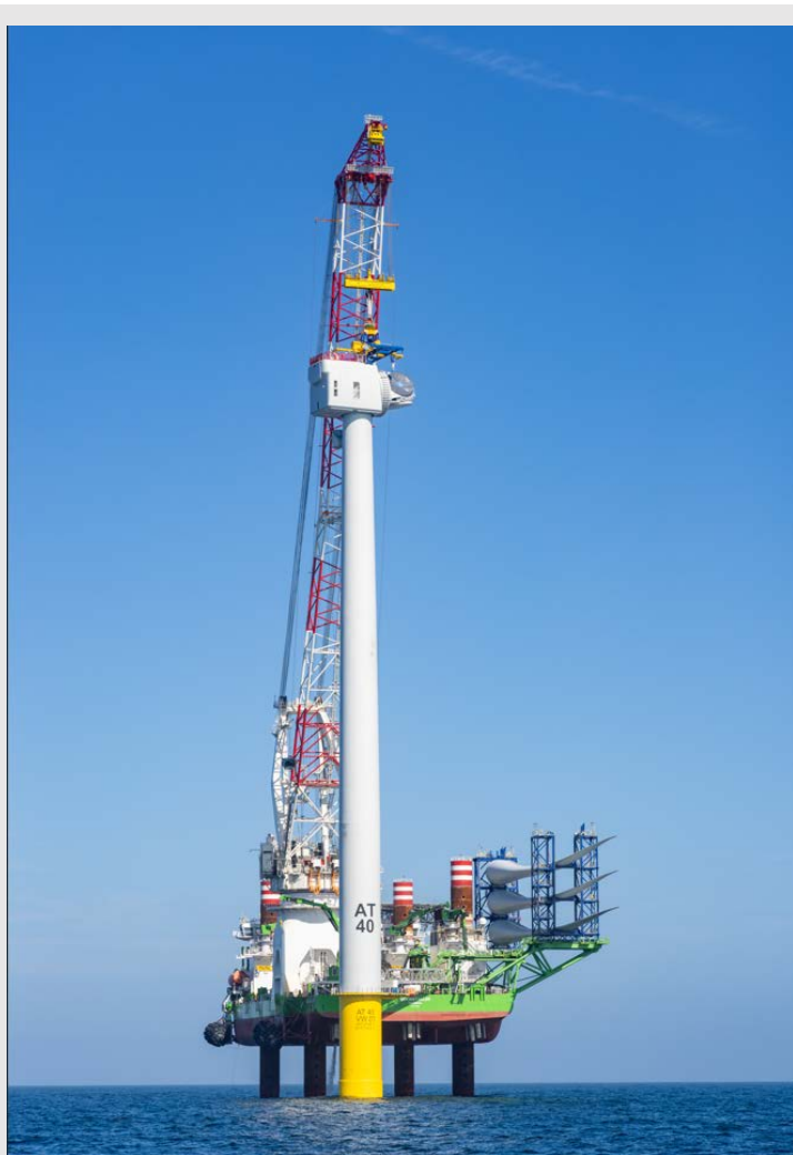
Vineyard Wind is the first utility-scale offshore wind energy project in the United States and sits over 15 miles off the coast of Massachusetts. Cybersecurity is an important consideration for new facilities to generate reliable, clean renewable energy. Photo by Joe DeNero, NREL
