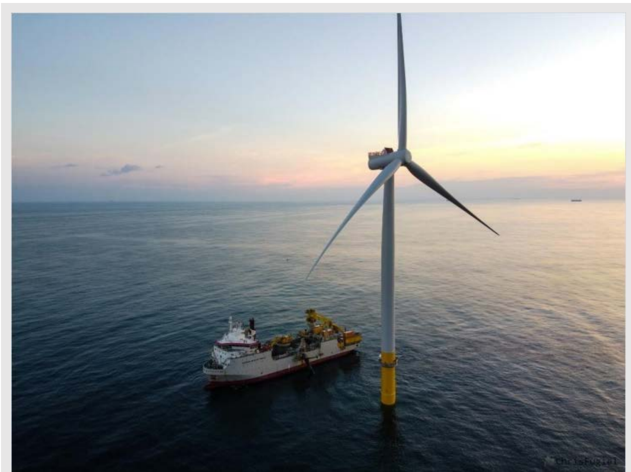
The Operations and Maintenance Roadmap for U.S. Offshore Wind Energy outlines ways the domestic offshore wind energy industry could improve operations and maintenance practices. Photo from Lyfted Media for Dominion Energy
