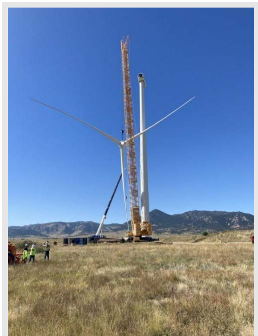
After 12 years of controls, drivetrain, and grid integration research, the Siemens Gamesa Renewable Energy 2-MW G97 wind turbine was removed from NREL's Flatirons Campus. Photo by Jeroen van Dam, NREL
