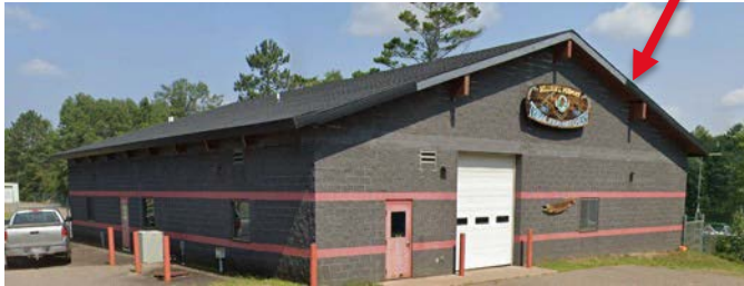
Potential solar PV array location #12; the red arrow points to the north-facing rooftop on the hatchery building for the array studied in this example. Image from Google Earth
