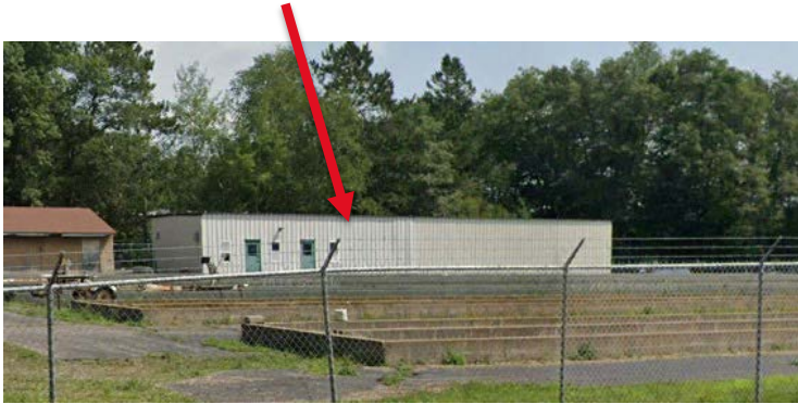
Potential solar PV array location #8. The red arrow points to the roof for the array. Image from Google Earth
