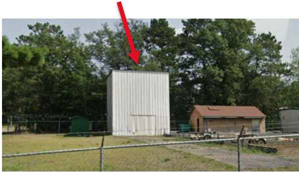
Potential solar PV array location #7. The red arrow points to the roof for the array. Image from Google Earth
