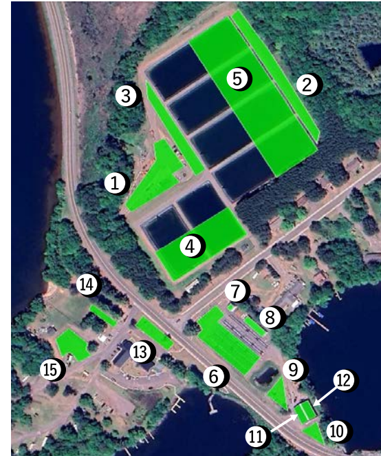
Locations identified by Lac du Flambeau staff for potential solar PV installations. Image from Google Earth
