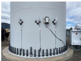
Three thermal cameras (AXIS Q1941-E Thermal Network Camera). Each sensor was mounted 70.25 inches off the ground/up the turbine and were 37.5 inches apart, pointing up at the blade. All recordings were collected with matching timestamps using a GPS module.
