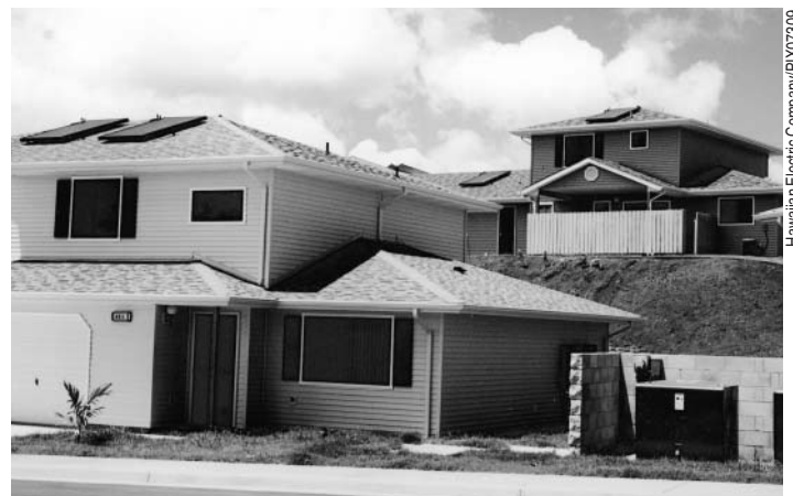
Each solar water-heating system at the Navy’s Moanalua Terrace housing project offsets about 1.7 tons (1.5 metric tons) of carbon dioxide, 8.2 pounds (3.7 kilograms) of sulphur dioxide, and 11.2 pounds (5 kilograms) of nitrogen oxide every year.
