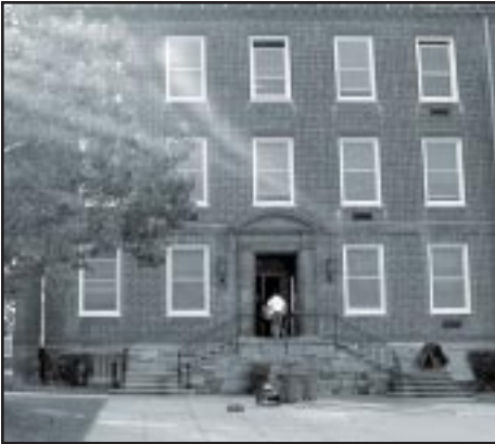
Washington, DC public schools partner with Rebuild America to implement energy efficiency improvements.
