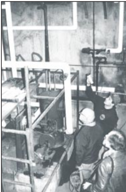
Rebuild Boston assesses existing systems and equipment and suggests areas for potential energy savings.
