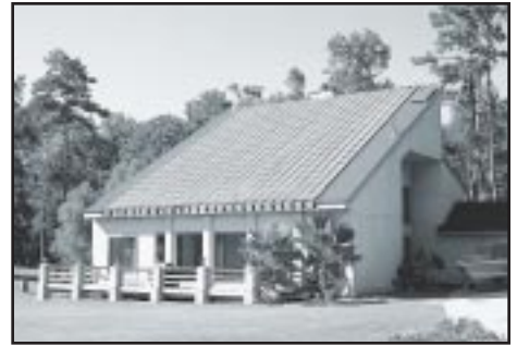
This home employs integrated solar roof panels.
