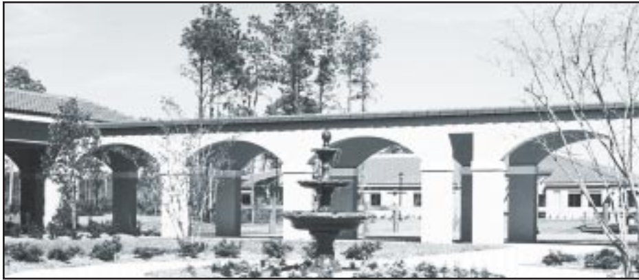
St. Johns River Community College in Florida reduced operating costs by implementing energy efficiency measures.
