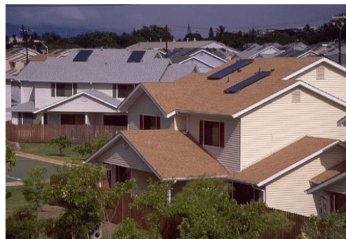
Fig. 1: Solar hot water systems installed on residences in the Navy's Moanalua Terrace family housing project.
