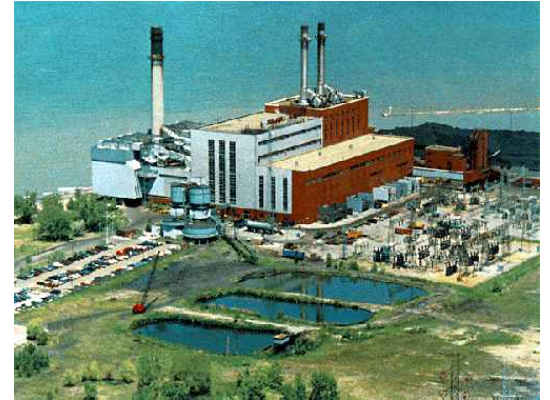
The Dunkirk Power Station will use hybrid willow grown by New York farmers to generate renewable electricity
