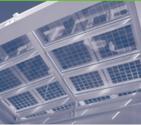
NREL/PIX 01082, LAWRENCE BERKELEY NATIONAL LABORATORY
