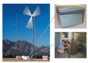
Hybrid power plants can use renewable energy to produce and store hydrogen on site. The hydrogen can then be used for transportation or by fuel cells to generate electricity when the wind isn't blowing. Such systems overcome the intermittency of solar and wind resources.
