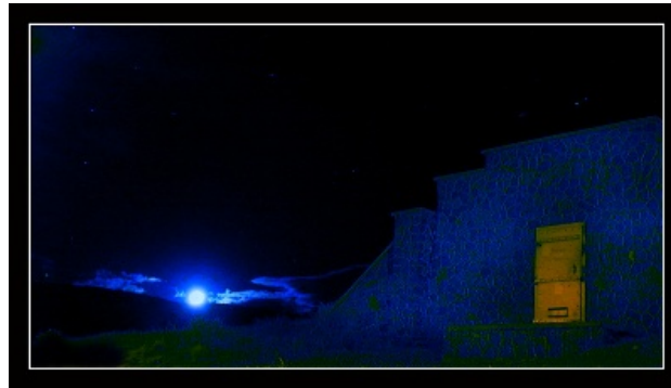
Figure 5.18. STM cultural resource. Stone and concrete ammunition bunker at STM. Photo courtesy of Stephen Wilcox.
