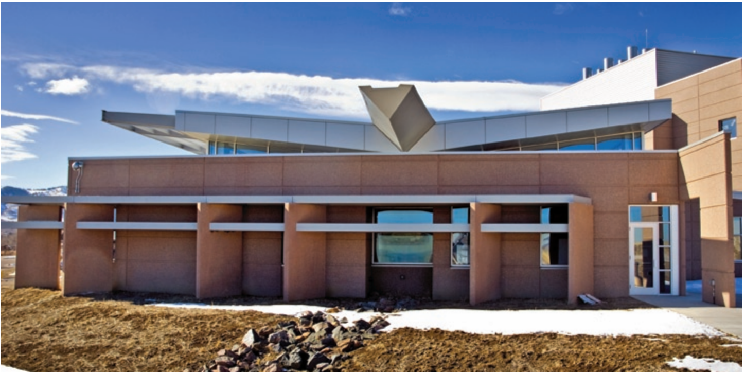
The roof of the Science and Technology Facility is designed to collect and direct rain water to irrigate the surrounding landscape.
