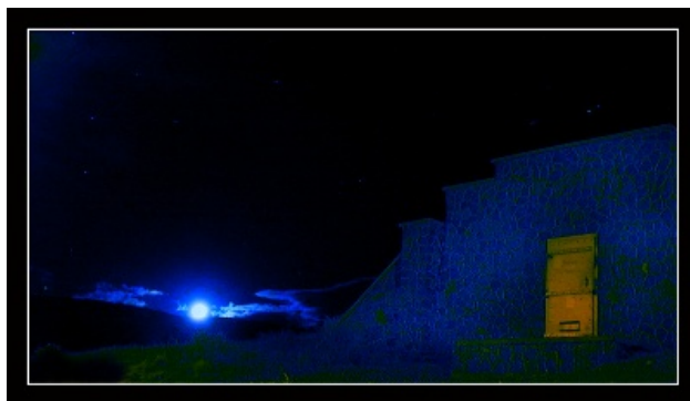
Figure 5.14. STM cultural resource: stone and concrete ammunition bunker at the STM
