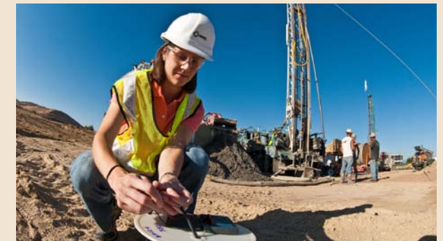
NREL senior geothermal analyst Erin Anderson examines a heat sensor that descends 500 feet under the IKEA store construction site in Centennial, Colorado. Photo by Pat Corkery, NREL/PIX 17906
