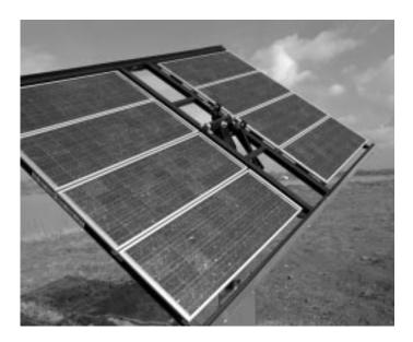
Crystalline silicon technology uses wafers similar to computer chips. Thin film photovoltaic cells use very thin layers of semiconductor material. While not as efficient as crystalline silicon cells, thin film cells use 30 to 100 times less semiconductor material and are easier and less expensive to make. NREL performs research in both areas.
