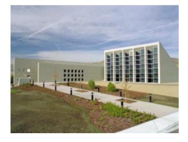
On the other side of the "V" is a thick concrete wall coated with black paint and faced with glass. A small airspace separates the wall from the glass. Direct solar radiation is absorbed by the wall, trapped by the glass and conducted inward to gradually heat the exhibit hall.
