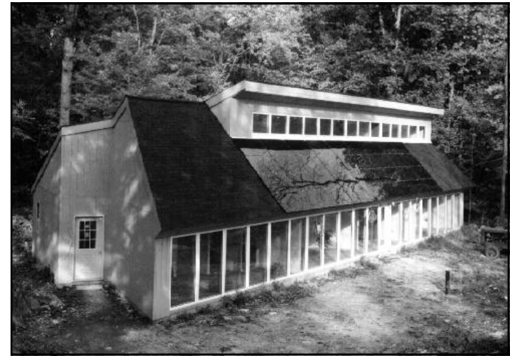
This utility-independent home in New Jersey is powered by a 1.8-kW p photovoltaic array.
