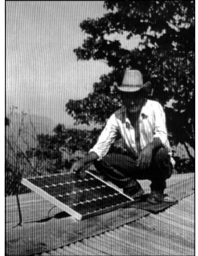
This Honduran farmer's PV system powers four lamps, a radio and a television. With technical assistance from Enersol Associates, Inc., an international nonprofit organization, a local coffee cooperative installed 100 such systems in 1994. By replacing polluting kerosene lamps, each PV system will eliminate 3-6 tons of greenhouse gases over its 20-year life. Enersol's solar-based rural electrification program in Honduras is supported in part by Sandia National Laboratories.
