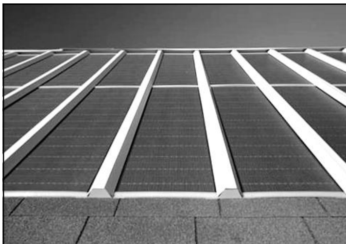
These roof-mounted PV panels replace conventional roofing shingles while supplying electricity to the building and the utility power grid.
