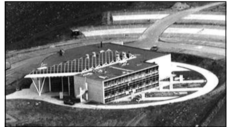
An aerial view of the Brundtland Center in Toftlund, Denmark. Opened in the summer of 1995, this high-tech office building makes use of several energy efficiency and renewable energy technologies, including the country's largest photovoltaic array. Semitransparent solar cells are integrated into the glass of the atrium roof, providing partial shading while producing 11,500 kWh of electricity at 220 volts AC.
