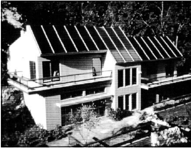
The Boston Edison "Impact 2000" home incorporates a 4-kW p utility-connected photovoltaic array.
