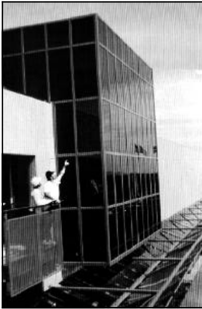
Thin-film photovoltaic modules used as exterior cladding on a factory facade
